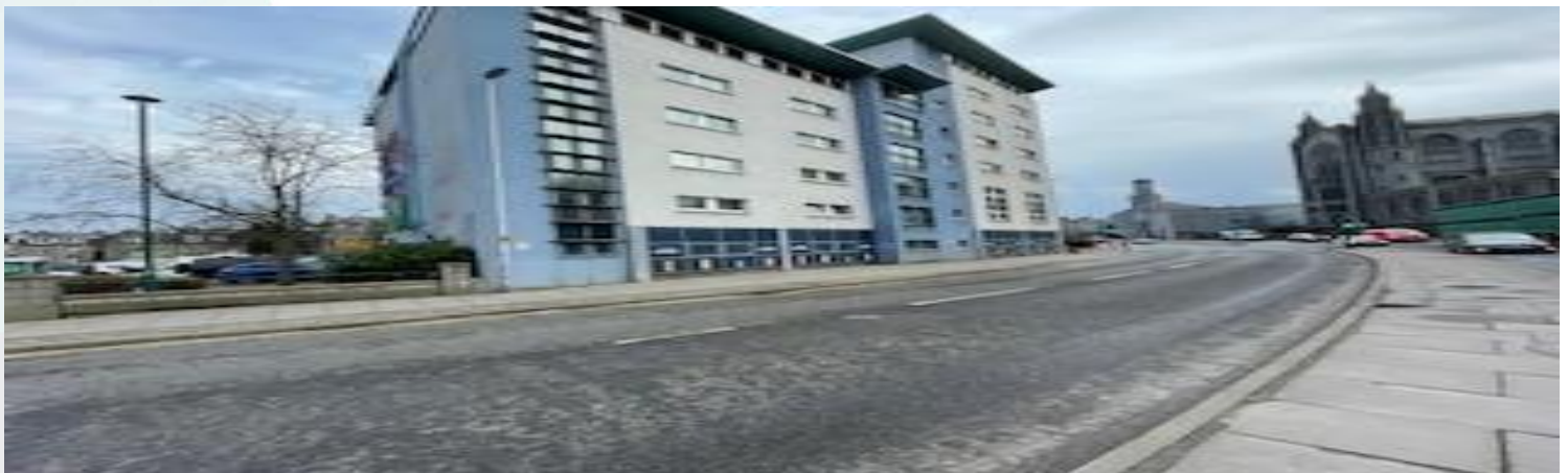
Phase 4 scaffolding lane closure and footpath restrictions.
