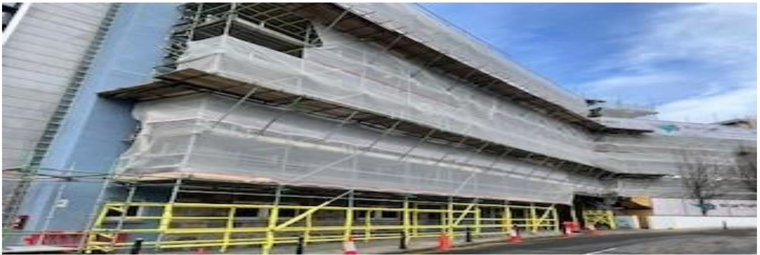
Phase 4 scaffolding front elevation
